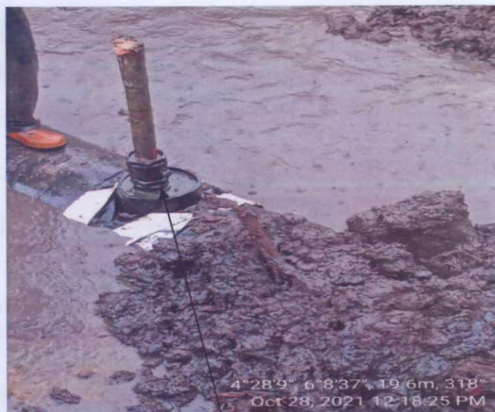
AFTER EXCAVATION (SPILL POINT)
